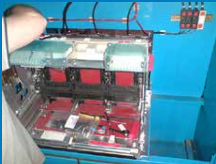
Direct Response Engineer Installing Retrofit ACB
